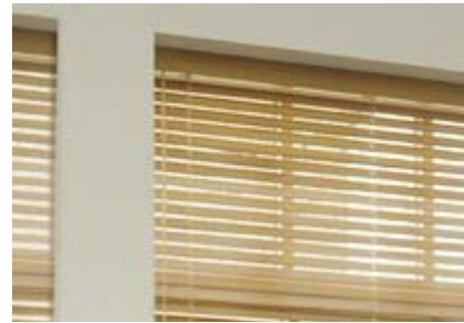
Suntracking : the tilt angle of the slats is set to protect the interior from direct sun irradiation while letting as much as possible daylight coming in
