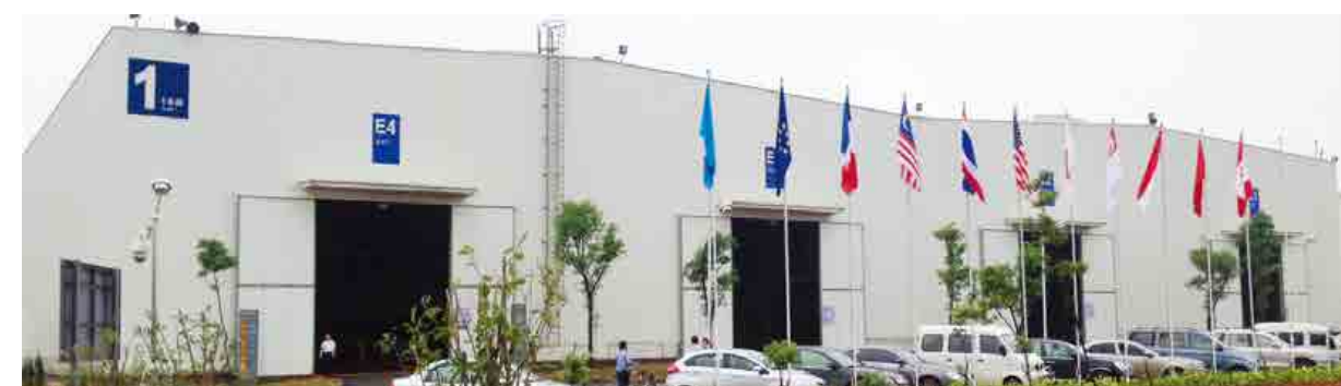
远大可建集团的白色厂房 White factory of Broad Sustainable Building Group
