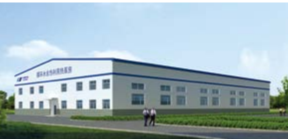
热泵房外部 Outside of heat pump house
