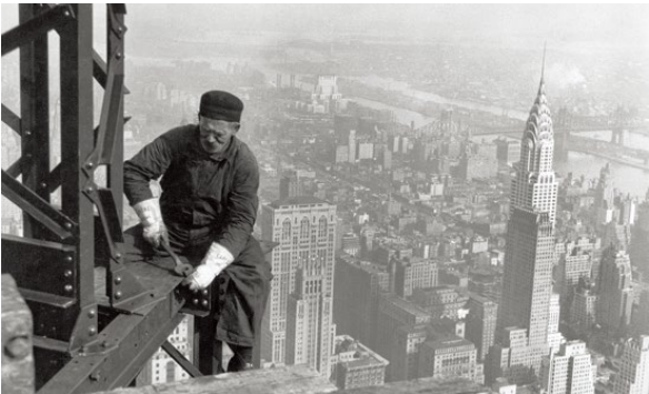
1930 年建的帝国大厦 The Empire State Building under construction in 1930
