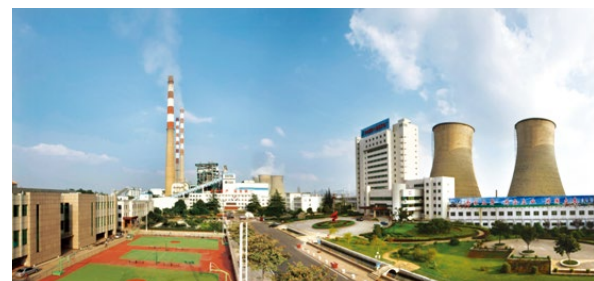
华电十里泉电厂 Huadian Shiliquan Power Plant
