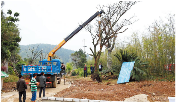
Ecological Afforestation of One-side Street after Removal
