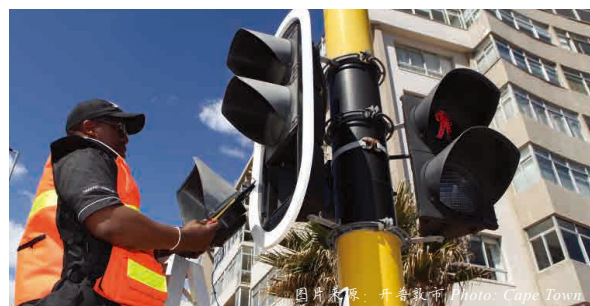
改造交通信号灯 Traffic lights being retrofitting
