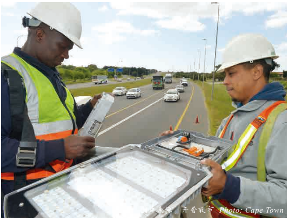
升级改造路灯 Retrofitting street lights
