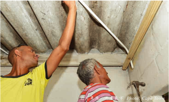
建筑屋顶翻新 Ceilings being retrofitted
