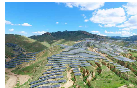
▲ 隆基股份建设的山西大同石仁村光伏扶贫电站 Shanxi Datong Shiren Village photovoltaic power station built by LONGi
