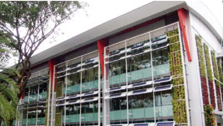
BCA Zero Energy Building
