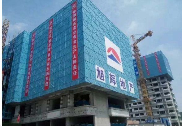
▲ 时代城项目工地实景 Real Site View of Times city
