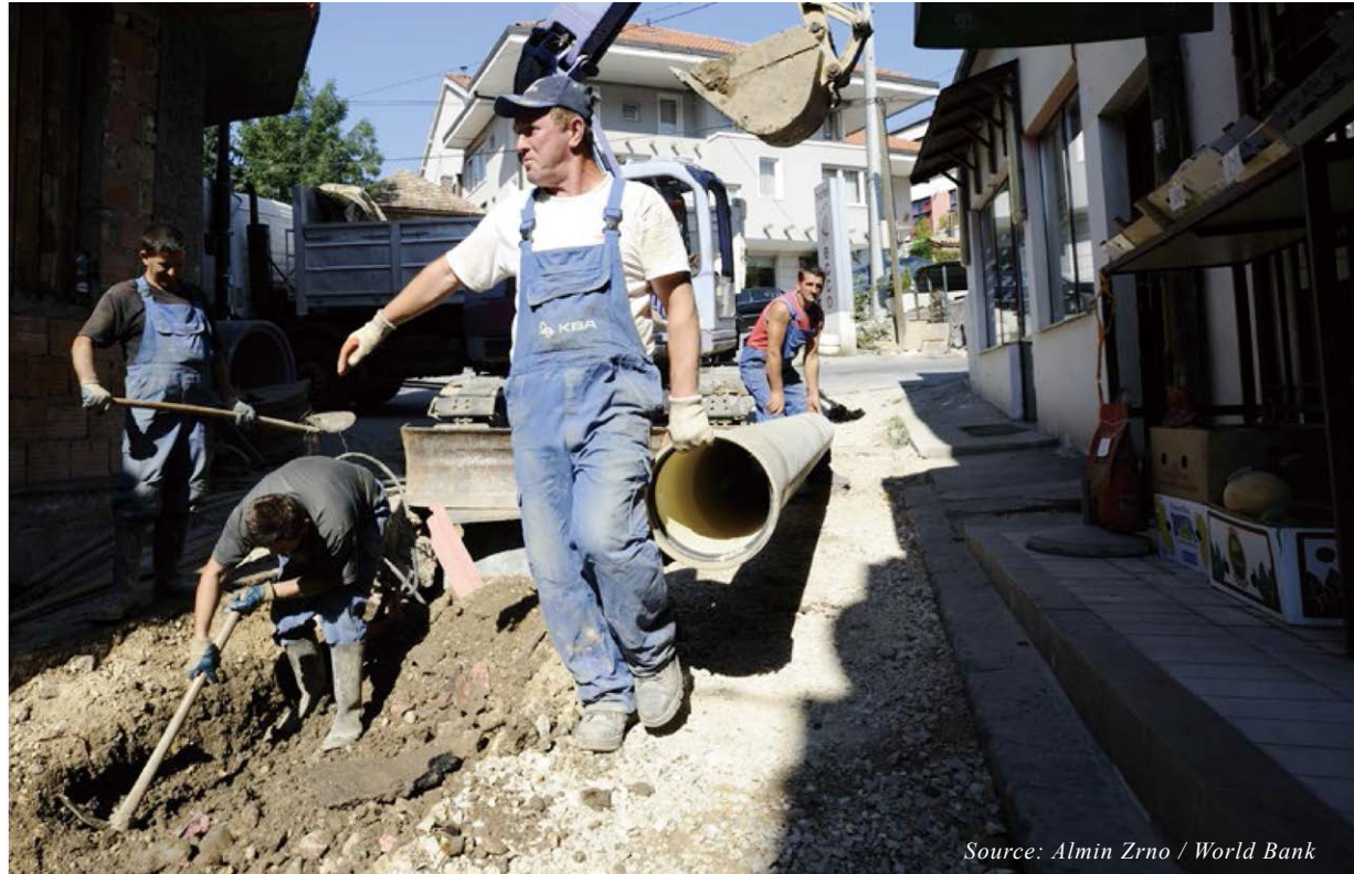
萨拉热窝市的工人正在维护废水网 Repair of waste water networks in Sarajevo
