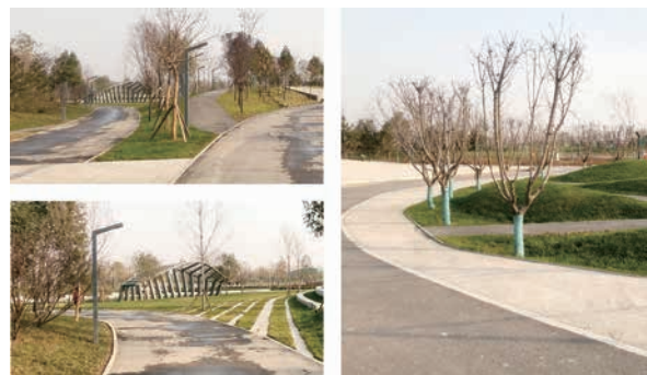
▲ 现场施工图 photo of site construction
