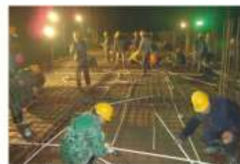
In August, 2009, the scene of constructing in Shuimo School, where the workers were working hard day and night
